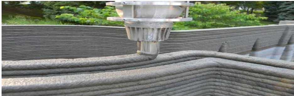
Figure 5. Layering of 3D Printable Concrete [9]
