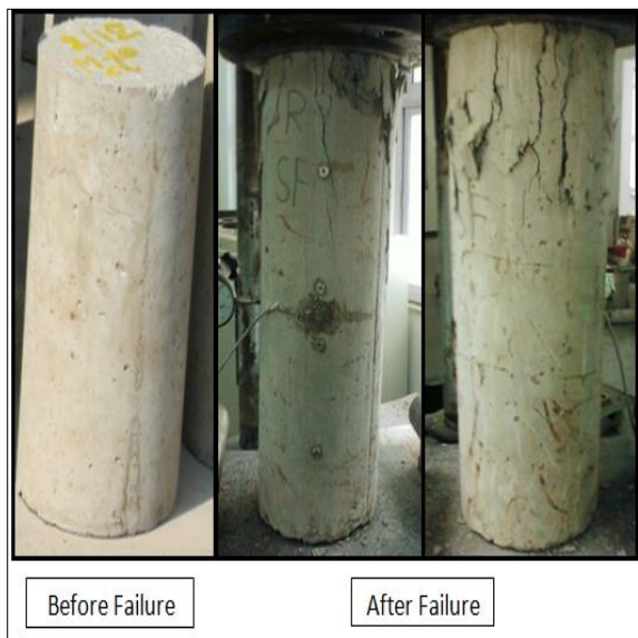
Figure 20 Crack patterns and failure mode of HSFRC
