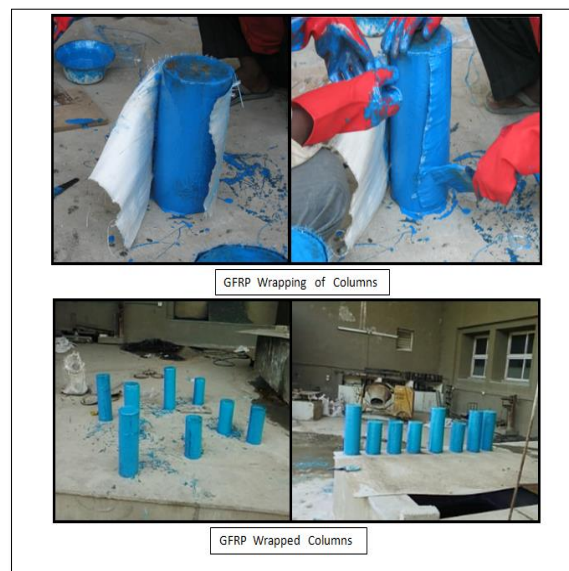
Figure 5 Application of GFRP sheet
