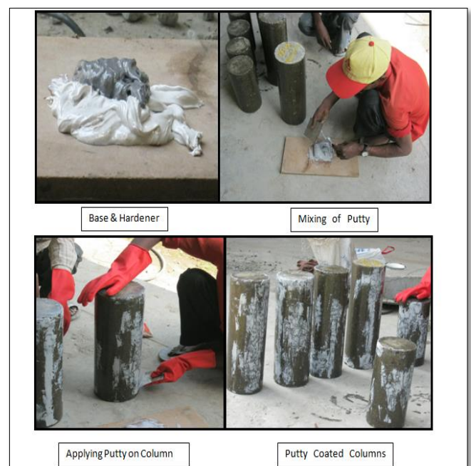
Figure 2 Application of putty on Column.
