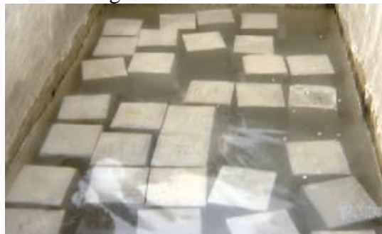
Fig.4.1.3. Curing of Concrete
