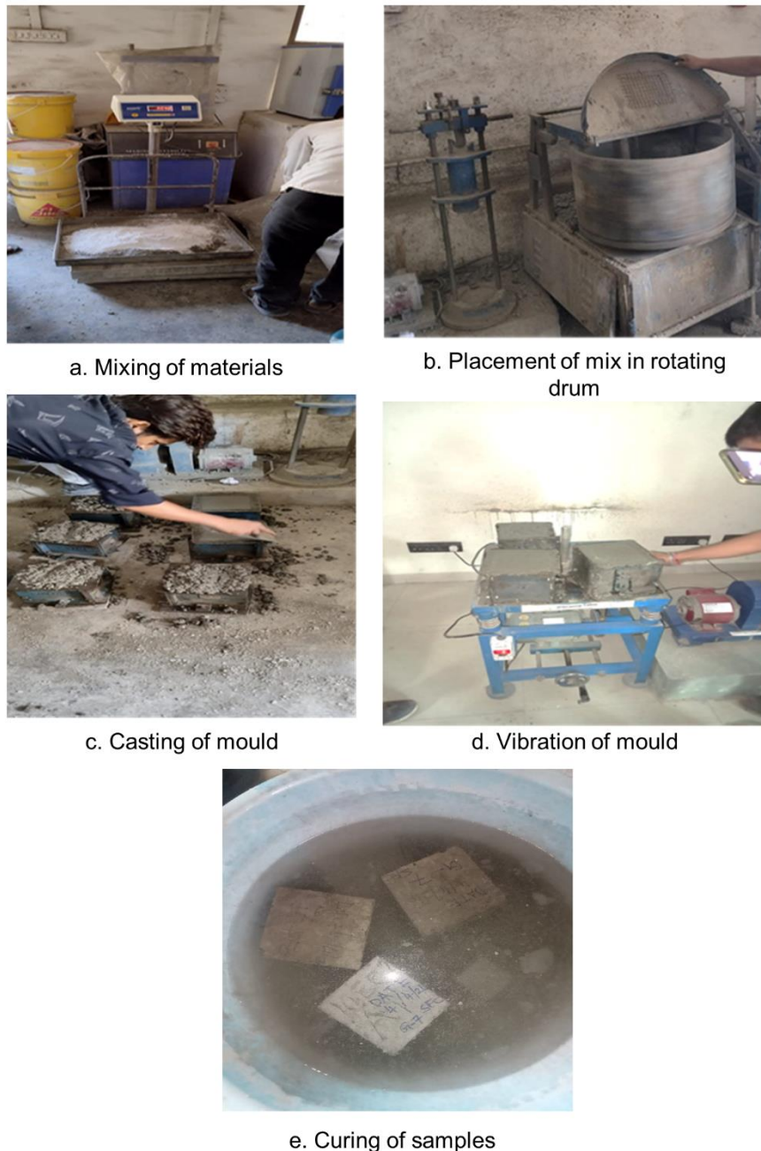
Figure 4. Various stages involved in study from of mix preparation to curing
