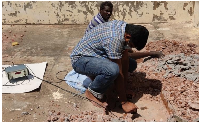
Figure 4. Testing of the structure by ultrasonic sonic pulse velocity test method
