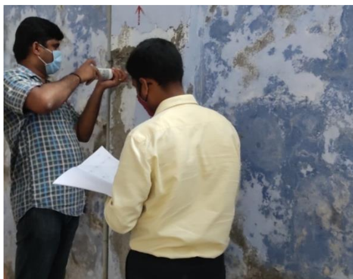
Figure 2. Testing of structure by rebound hammer test method
